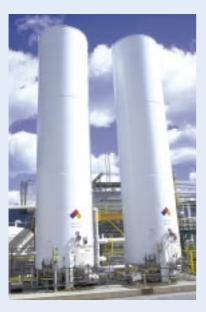
The Cash range of cryogenic products are used predominantly on cryogenic gas systems. Many industrial gas supply companies now supply their gas in its liquefied state. In this context the term "cryogenics" is the liquefaction of gases. Typically the liquid is then turned back to a gas on site, whenever demand is generated.
